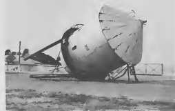
Looking like a rocket ready to be launched into space is Tank # 301 until recently in service at Powerhouse # 2 as a boiler water reservoir. The tank has been taken down for dismantling after 31 years. Pareciendo un raketa cla pa ser lanzá den espacio ta Tank # 301, te recientemente den servicio na Powerhouse # 2 como reservoi pa awa pa boiler. E tanki a ser bahá pa ser kibrá despues di 31 anja.
